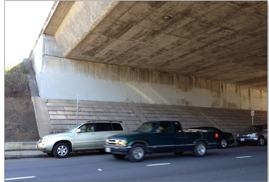
FIGURE 4.10 Concrete support wall opposite from site on South 3 rd Street
