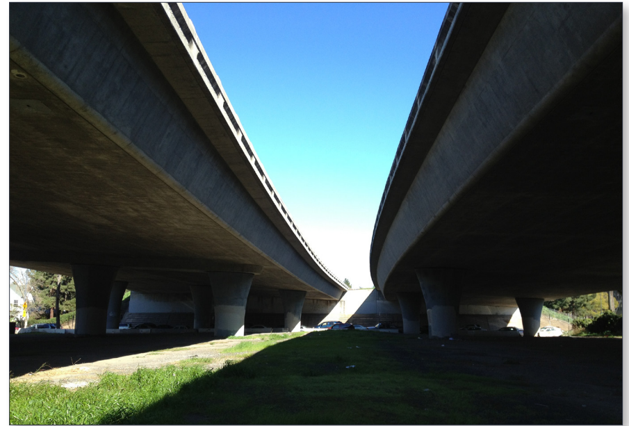
FIGURE 4.8 Gap in the freeway deck above the study area
