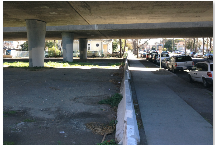
FIGURE 4.4 View of existing streetscape off of South 2nd Street
