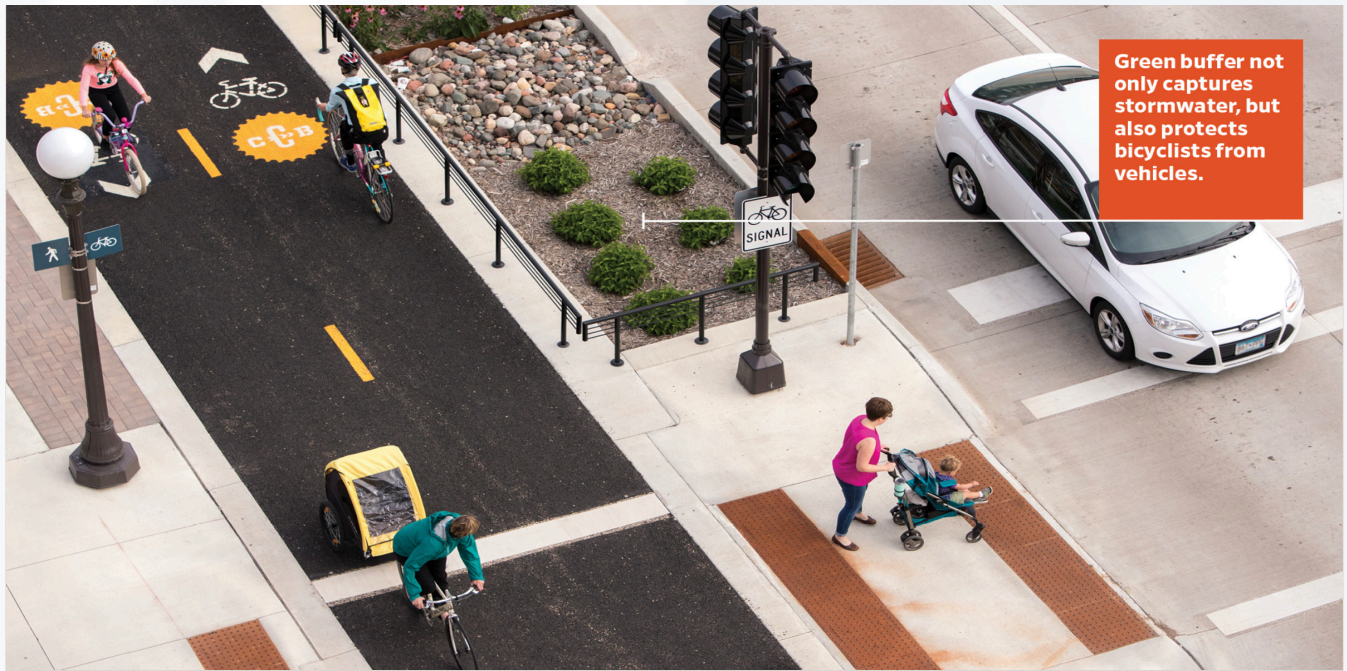
Figure 17: Jackson Street Reconstruction Project.
