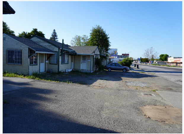
Figure 28: Existing condition of Burbank
