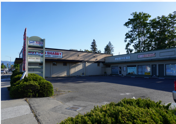
Figure 30: Existing condition of Burbank.
