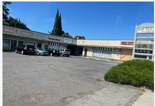
Figure 31: Existing condition of Burbank
