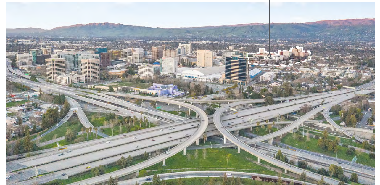
The Downtown San José skyline looking northeastward from the interchange of I-280 and SR-87.
